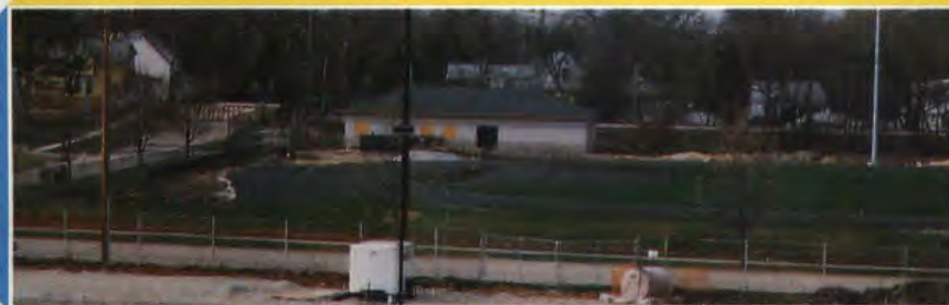
The new eight lane track and concession stand sit just across the street from where the old track used to be.
